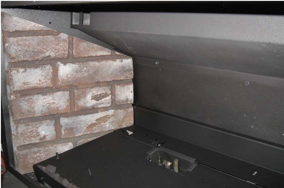
Left Brick Panel Placement as Shown
